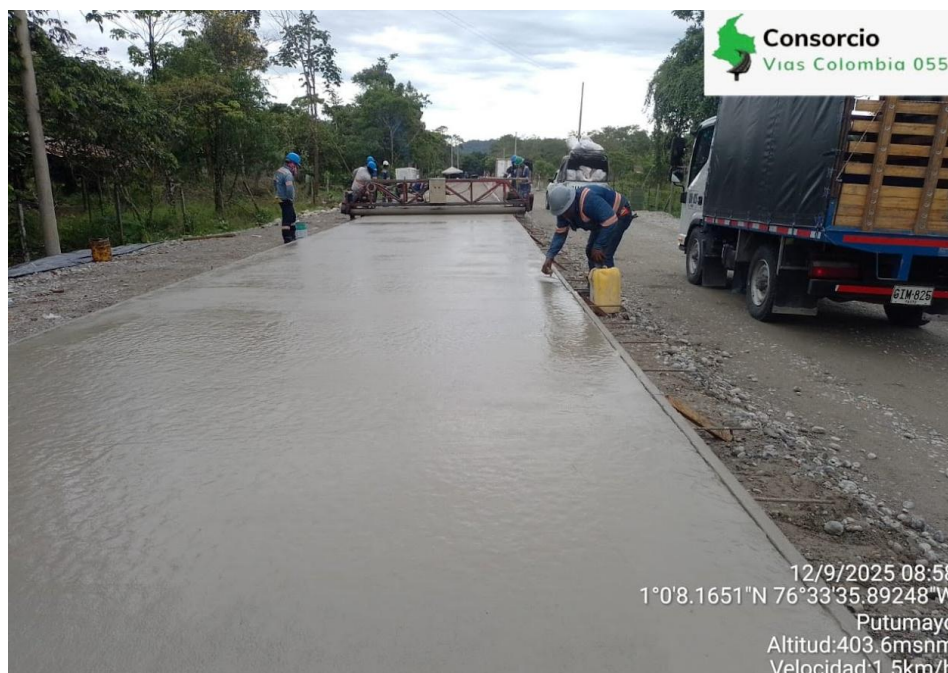
Figura 9. Fundida Concreto MR 45 PR 7+900.
