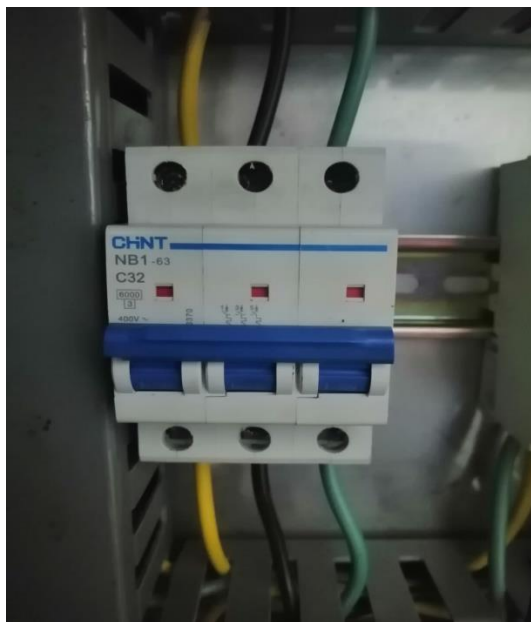
Figura 6-2. Disyuntor NB1 – 63 C32
