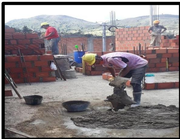
**Figura 49: Mezclado de mortero en obra.**
