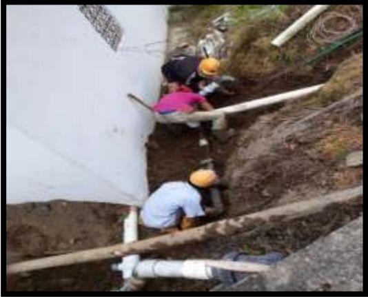
A photograph showing several workers in a trench installing large white PVC pipes. One worker in a blue shirt and yellow helmet is in the foreground, while others are visible further down the trench. The trench is dug into the earth, and a white tarp is partially visible on the left side. |
