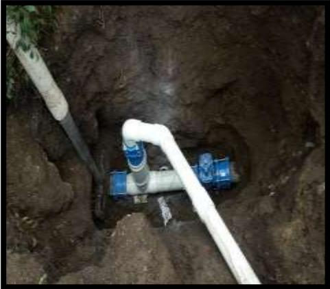
A close-up photograph of a baypass system installed in a trench. It features a blue valve and a white pipe that bypasses a section of the main pipe. The trench walls are dark and rocky.                                                                                                        |
