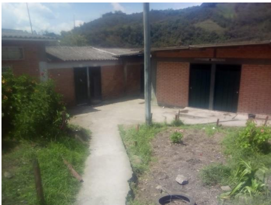
Figure 3: CER San Miguel bathrooms
