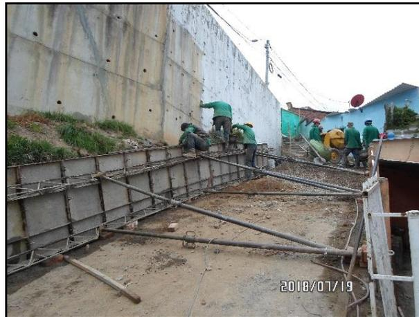
**Figura 23.** Muro concreto contención  $0 < h < 1.00$ mts.
