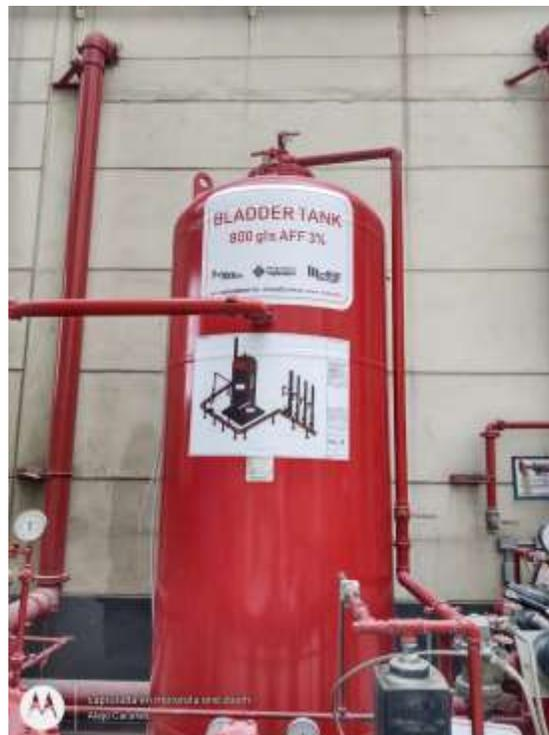
Figura 101. Caracterización Bladder tank. [ING FIRE]
