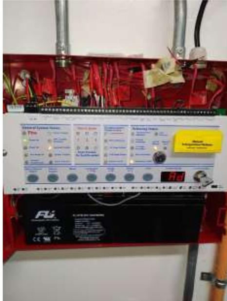
Figura 117. Panel de control agente limpio Toxement. [ING FIRE]
