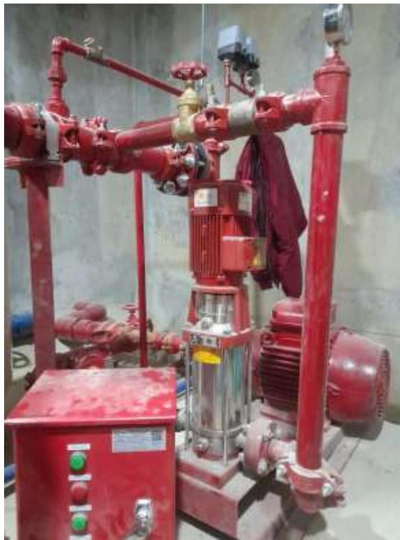
Figura 125. Panel bomba Jockey y motor bomba Jockey. [ING FIRE]
