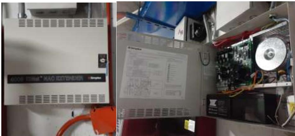
Figura 63. Fuente auxiliar 4009 NAC ID NET, instalada. [ING FIRE]
