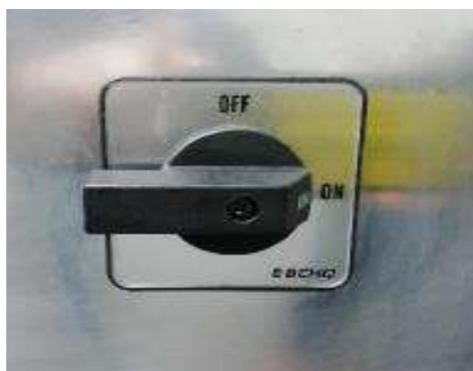
Figura. (7.11) 1: Selector principal en modo ON.
